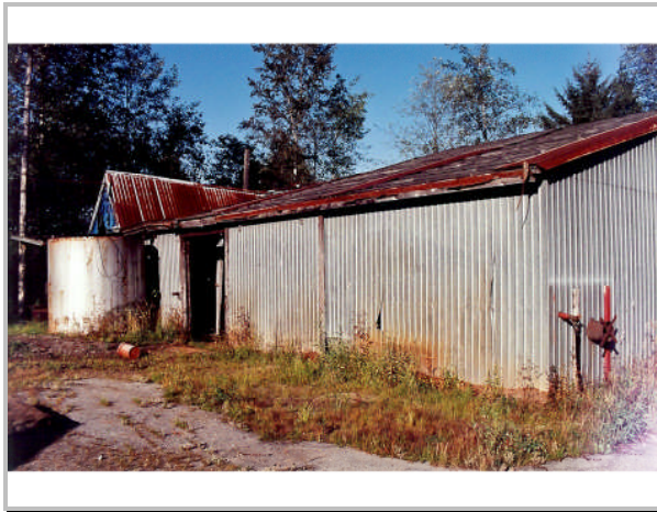
Langley Peat - the plant operation
